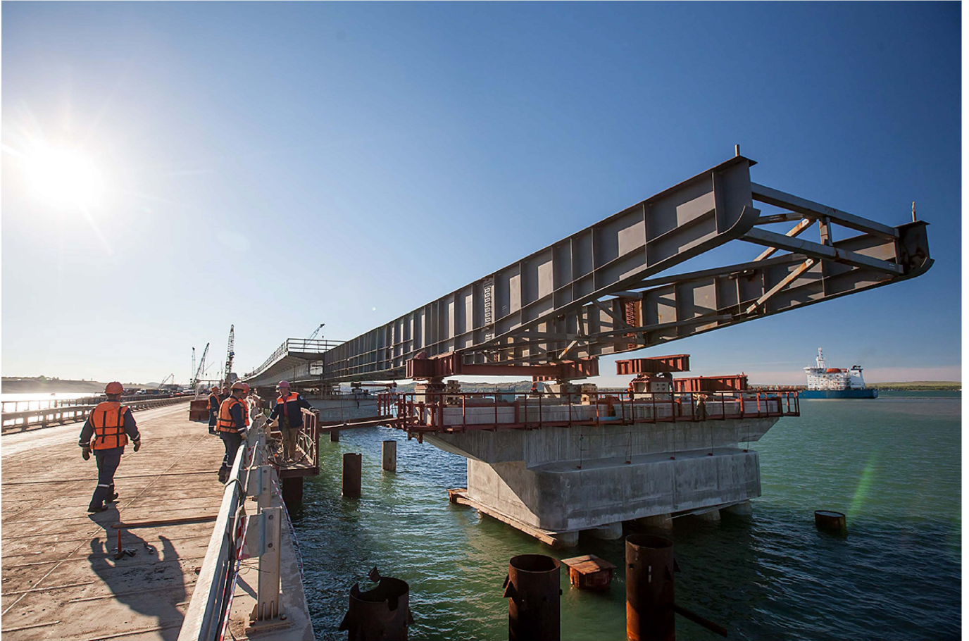
The lagging of sea spans of the road bridge, June 2017. Source: www.most.life
