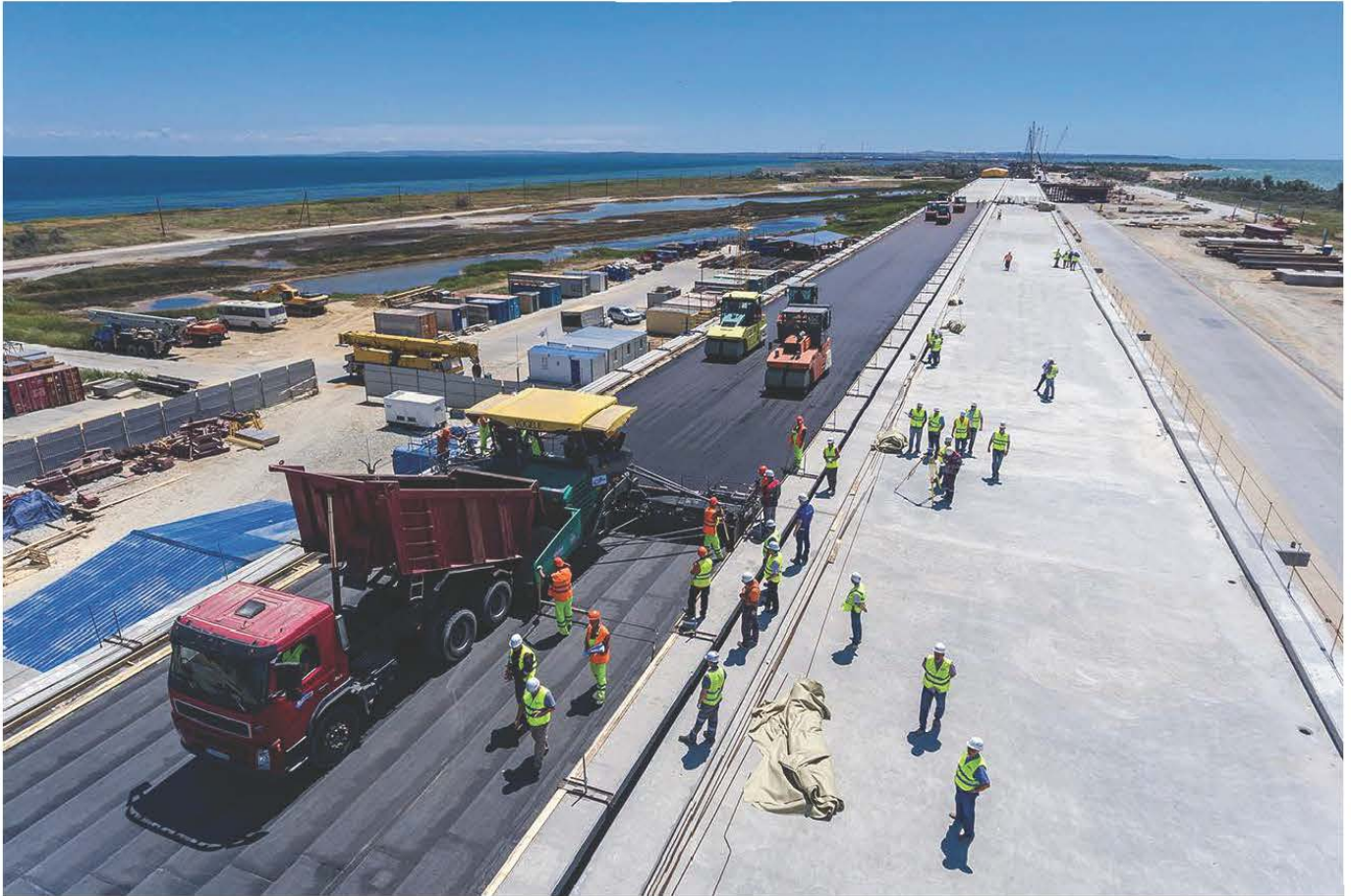
First asphalt placement. Source: www.most.life
